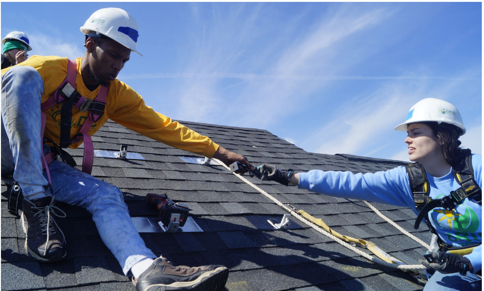
2019 Solar Works DC team in Northeast DC
