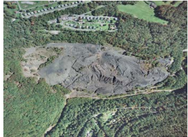
Typical coal refuse pile on abandoned mine lands. This site is Mine 37 located near Windber, PA along the Paint Creek.
