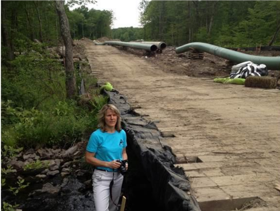
Delaware Riverkeeper Network Documents Pipeline Construction Activity in the Delaware River Basin
