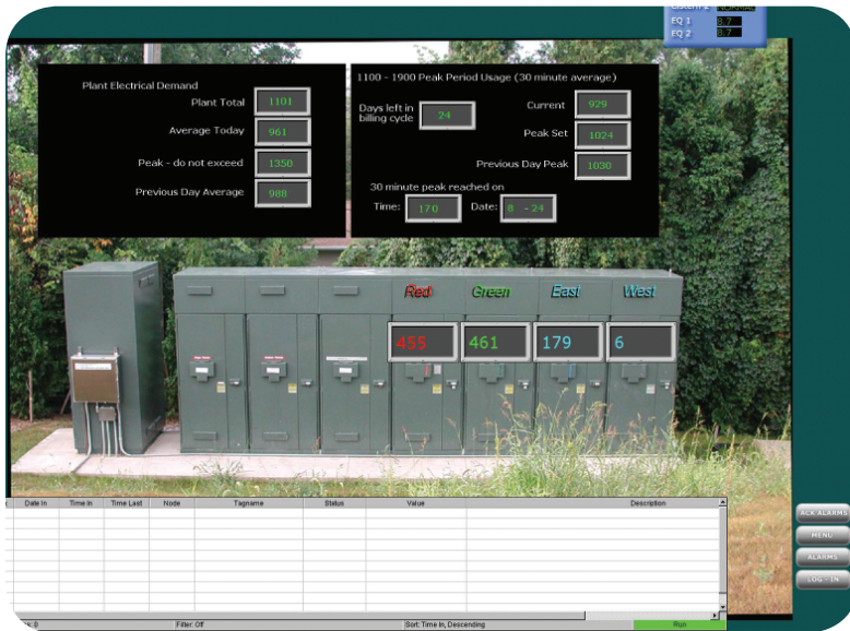
Ann Arbor invested in Rockwell Software RSPower Plus software and four Allen-Bradley PowerMonitor devices with Ethernet, which connect the devices to the process control network.
