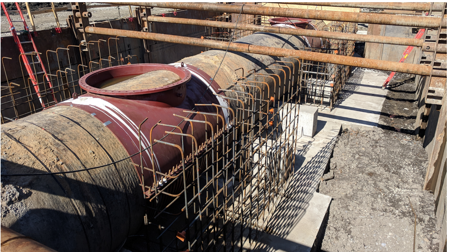
Construction on the Christina River Force Main that conveys wastewater to the Wilmington Water Pollution Control Facility in DE. Photo credit to Delaware Department of Natural Resources and Environment Control.
