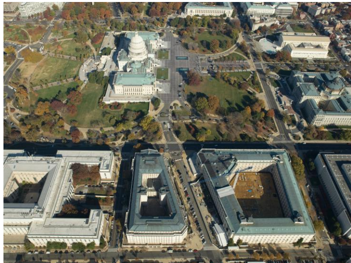
VIEW OF THE U.S. CAPITOL CAMPUS AND THE HOUSE OF REPRESENTATIVES BUILDINGS
