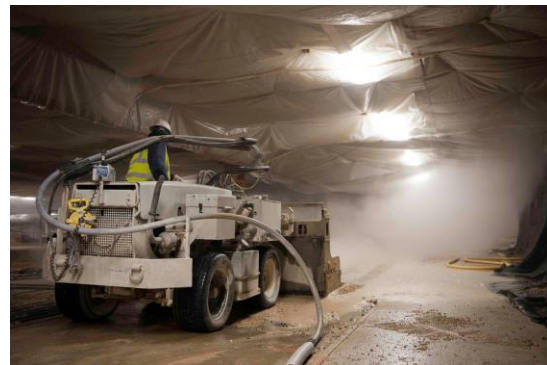
RAYBURN GARAGE REHABILITATION PROJECT
