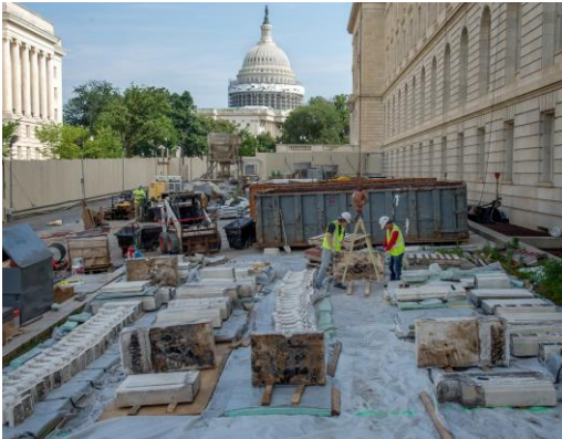
INITIAL PHASE OF THE CANNON RENEWAL PROJECT
