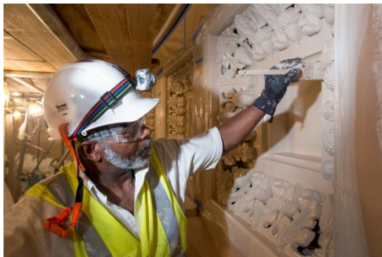
RESTORATION OF THE U.S. CAPITOL ROTUNDA
