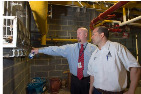
HOUSE EMPLOYEES MONITOR ENERGY USAGE BY INSPECTING STEAM EQUIPMENT
