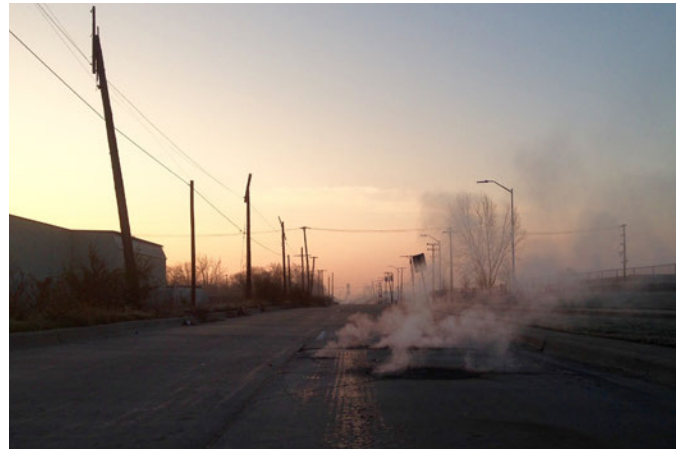
Steam is released along the steam loop displaying the inefficiency of the system.
