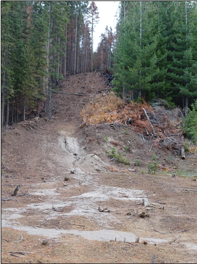
3(c)i Erosion from a steep dozerline Johnson Creek Fire, Idaho 2017. Photo credit: Friends of the Clearwater
