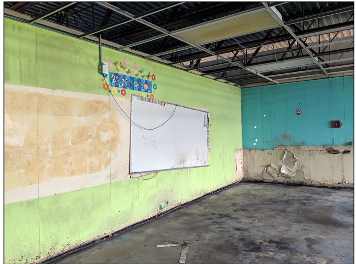
Classroom with molded floors and water damage on the walls at the Berwind Intermediate School in San Juan, Puerto Rico.
