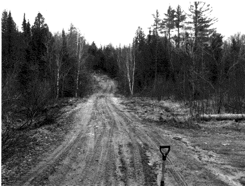
Attachment 7: Photo Along CR 595 Alignment
