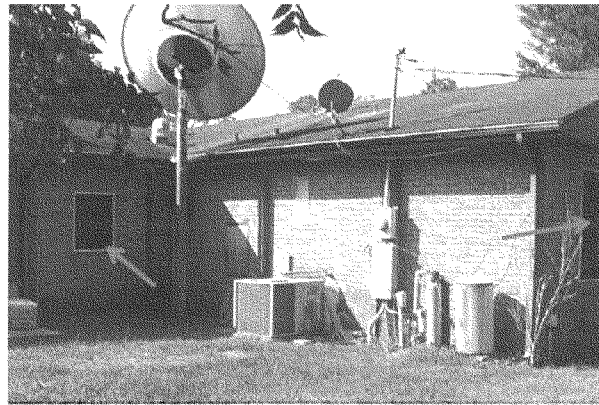
Solar Screens on North Side
