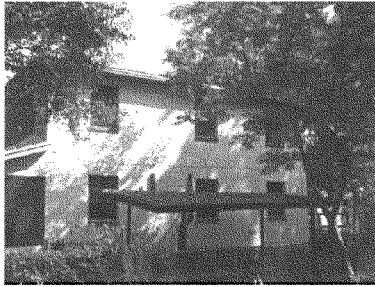
Solar screens installed on shaded West wall
