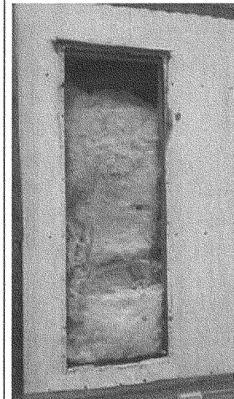
This is a picture of several batts of insulation jammed around the water heater.
