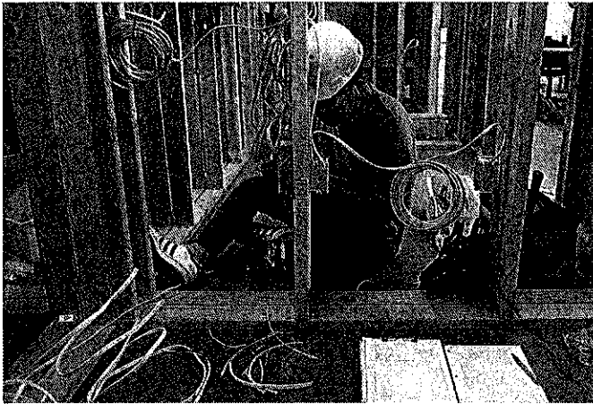
A student works on the wiring of an electrical outlet in Albuquerque, N.M. May, 26, 2021. PHOTO: ADOLPHE PIERRE-LOUIS/JOURNAL/ZUMA PRESS
