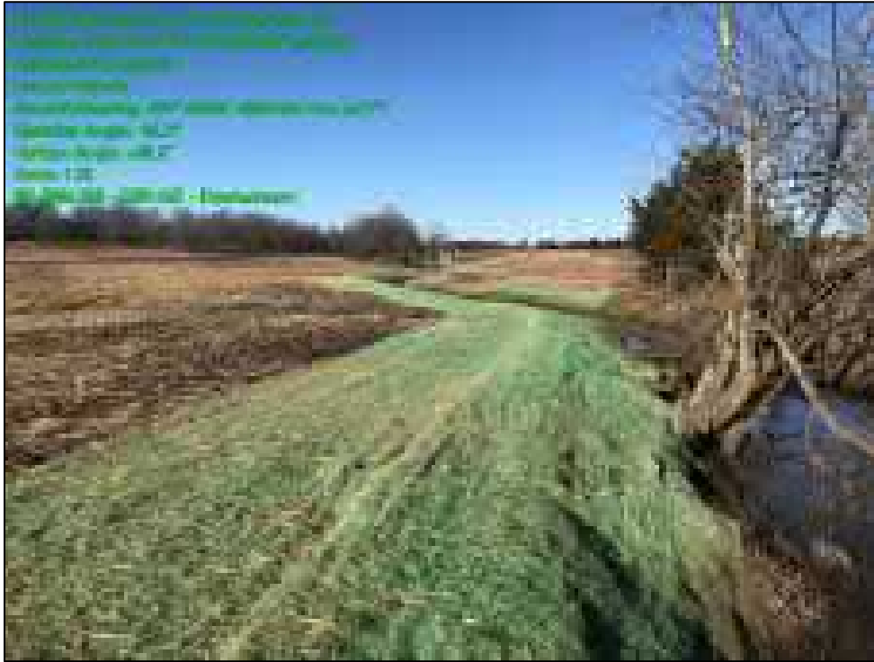
Downstream of Waterbody SBR-061 (S-BR-TAS-17/01/16-01) near MP 174.8 on 01/07/20 (Tract BR-0886.000).
