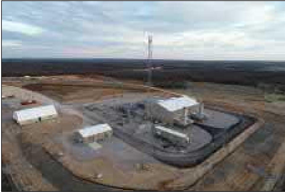
Aerial view of Tatums Compressor Station in February 2020.
