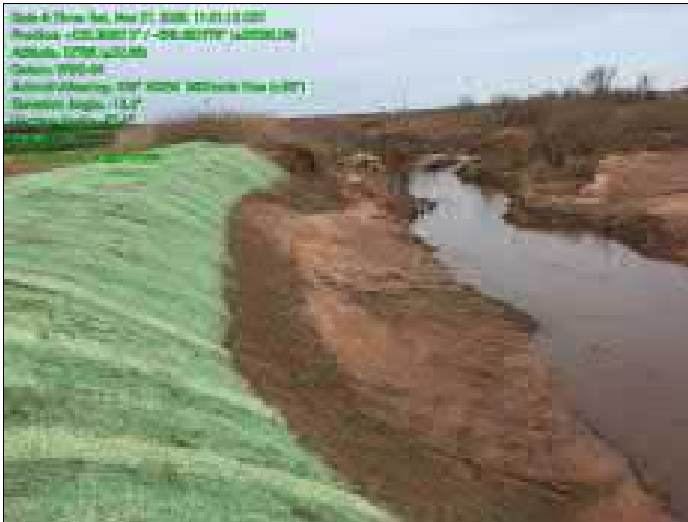
Upstream of Waterbody SCR-013 Buggy Creek (S-GR-RFT-16/12/10-1) near MP 34.8 on 03/21/20 (Tract GR-0132.010).
