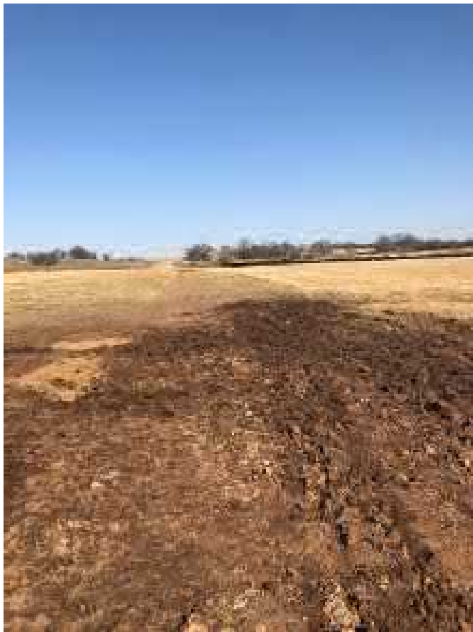
Midship Operations completed backfilling over Midship Pipeline on Nov 19, 2020
