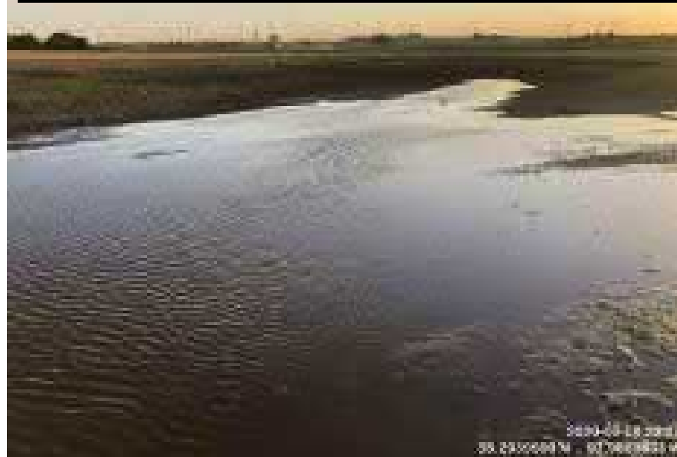
Bare Easement. Improperly Restored Drainage Causing Ponding On-ROW and Off-ROW
