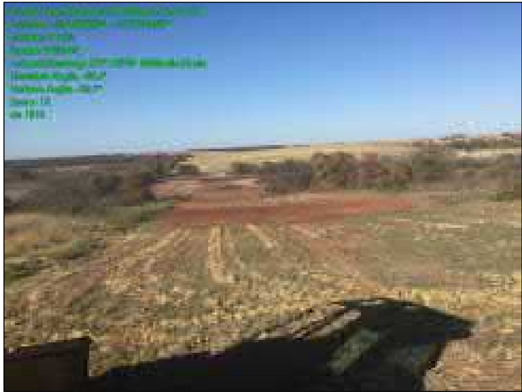
Maintenance work on Sandy Creek Farms property near MP 72.2 on 11/05/20.
