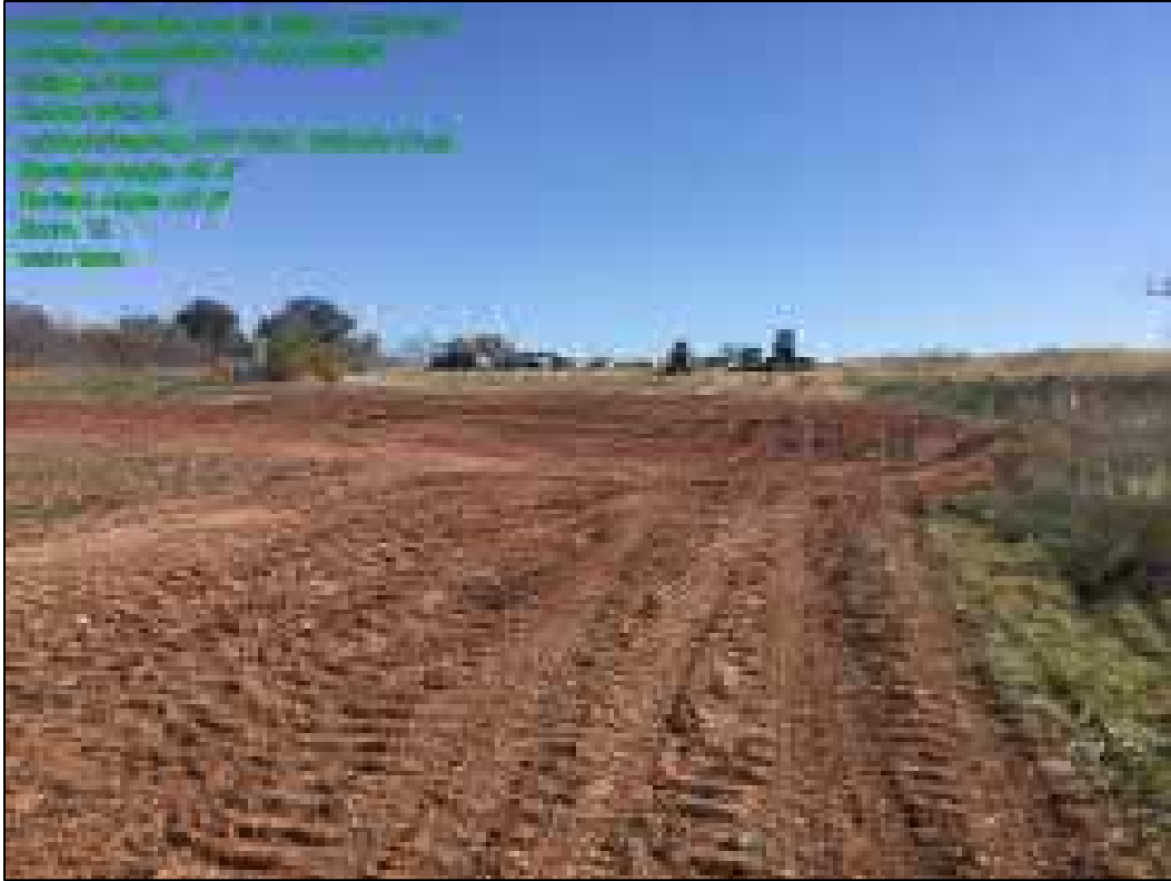
Maintenance work on Sandy Creek Farms property near MP 72.1 on 11/05/20.
