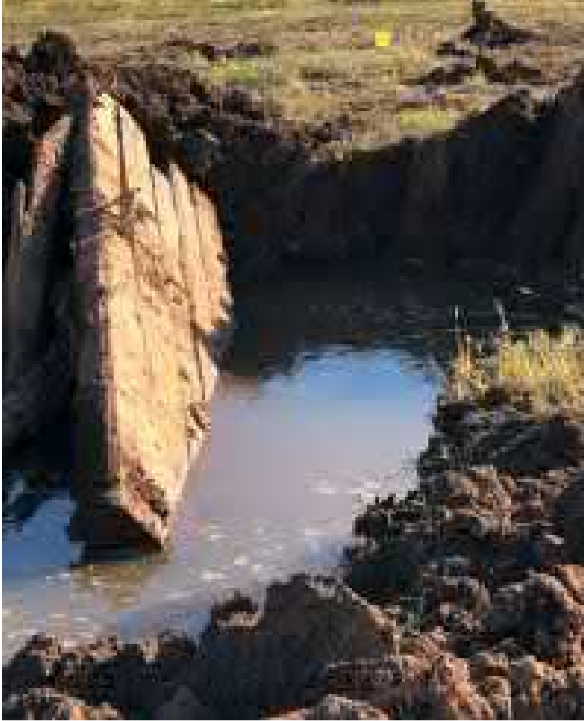
Excavations by landowner on Nov 18, 2020, mats located 4 – 4 feet below surface.
