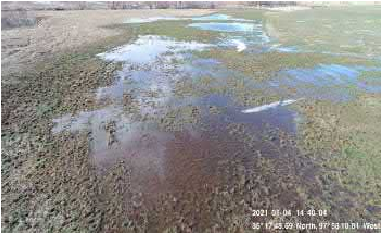
The Grade Has Not Been Restored Causing Ponding and Additional Compaction
