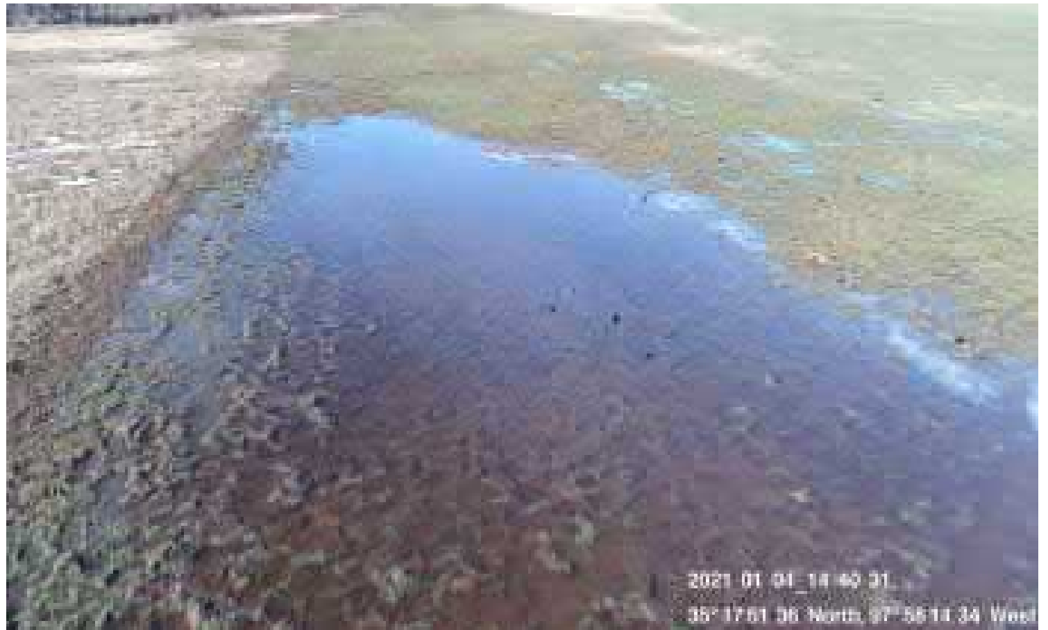
The Grade Has Not Been Restored Causing Ponding and Additional Compaction
