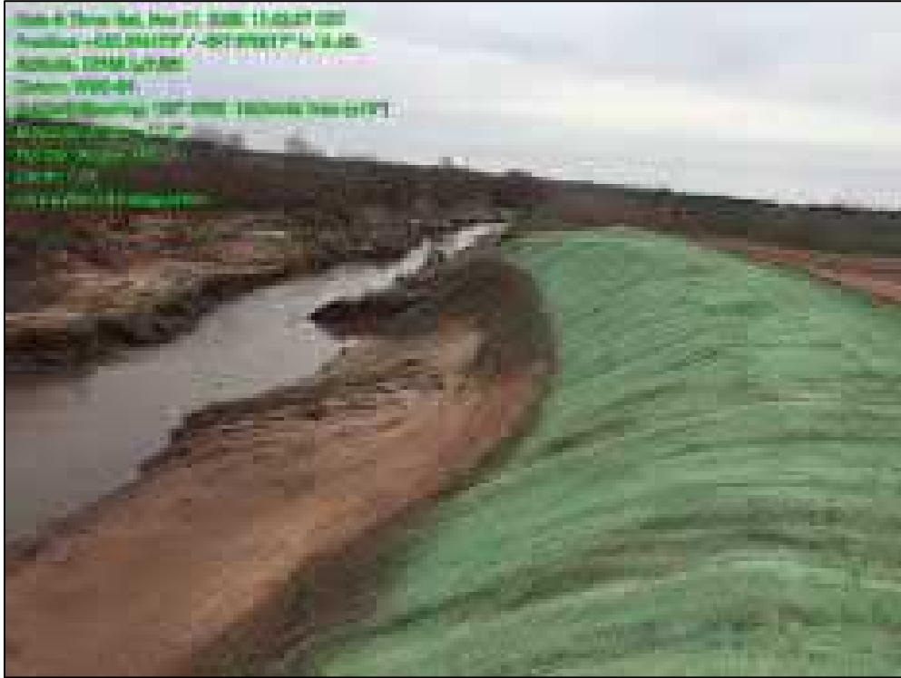
Downstream of Waterbody SCR-013 Buggy Creek (S-GR-RFT-16/12/10-1) near MP 34.8 on 03/21/20 (Tract GR-0132.010).
