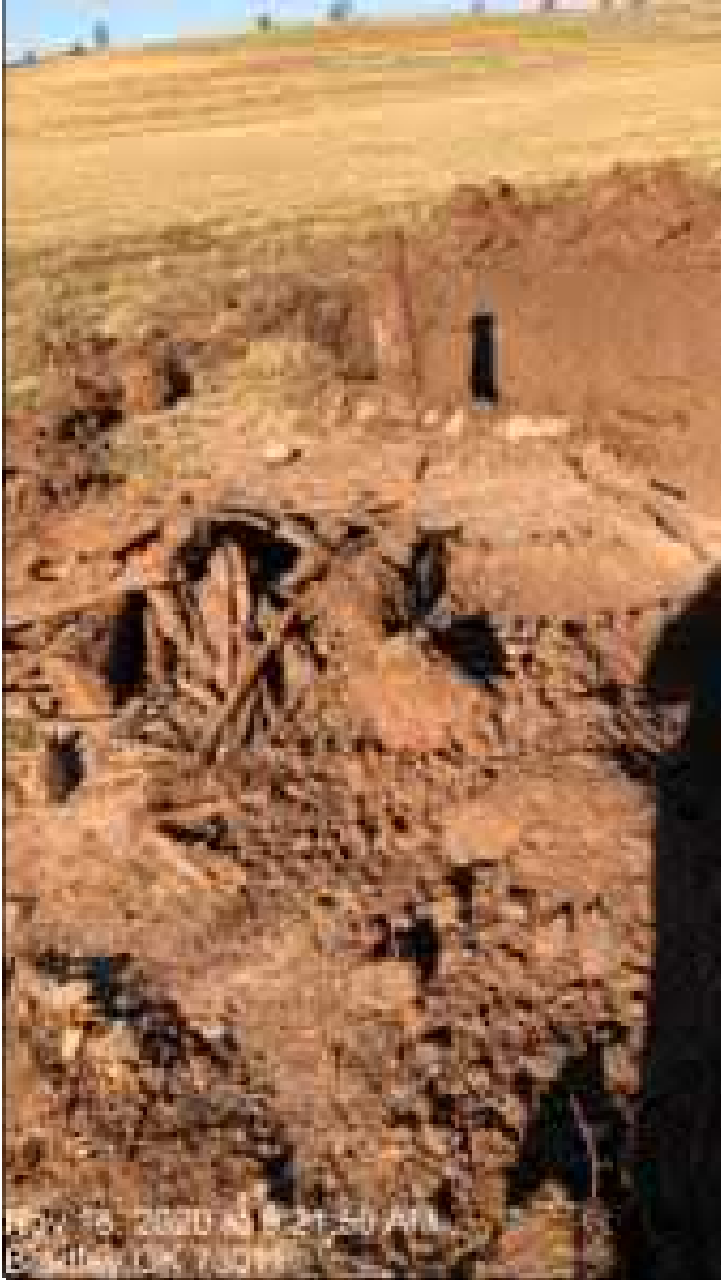
Excavations by landowner on Nov 18, 2020, construction debris located 4 – 6 feet below surface
