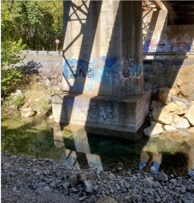
Figure 22: St. Mary's River Underneath Railroad Bridge
