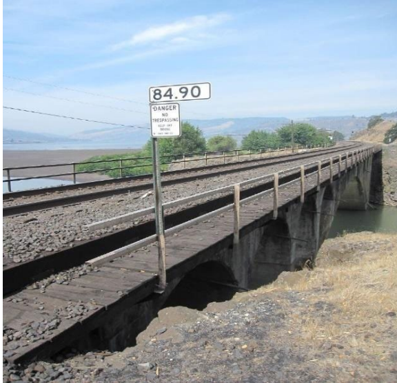
Figure 3: Coal at Klickitat River Bridge
