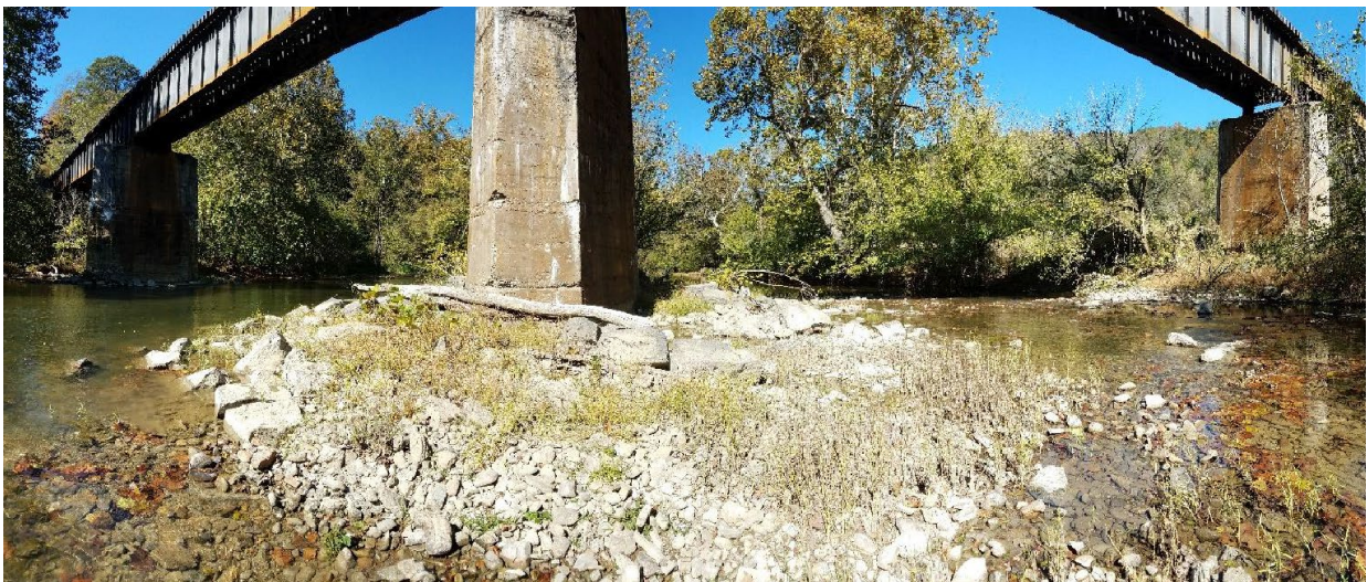
Figure 29: Photograph of Rail Bridge identified in Figure 28 over Clinch River
