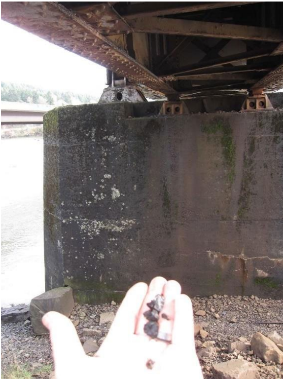
Figure 2: Coal Found Under BNSF Bridge at Confluence of Wind River and Columbia River
