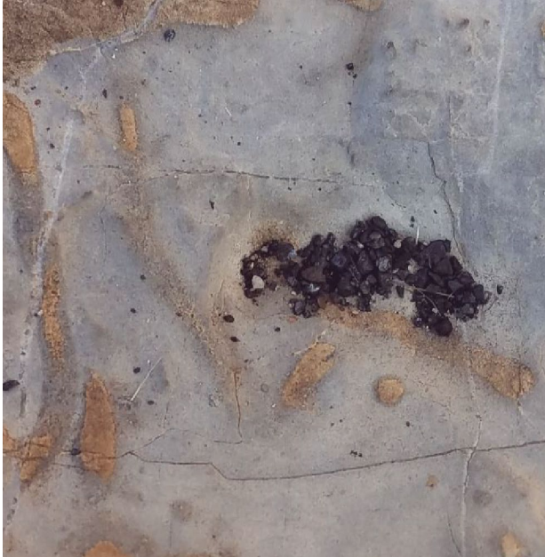
Figure 34: Coal Pieces that were Collected by Brush on Rock Located Next to Clinch River, under Railroad Bridge
