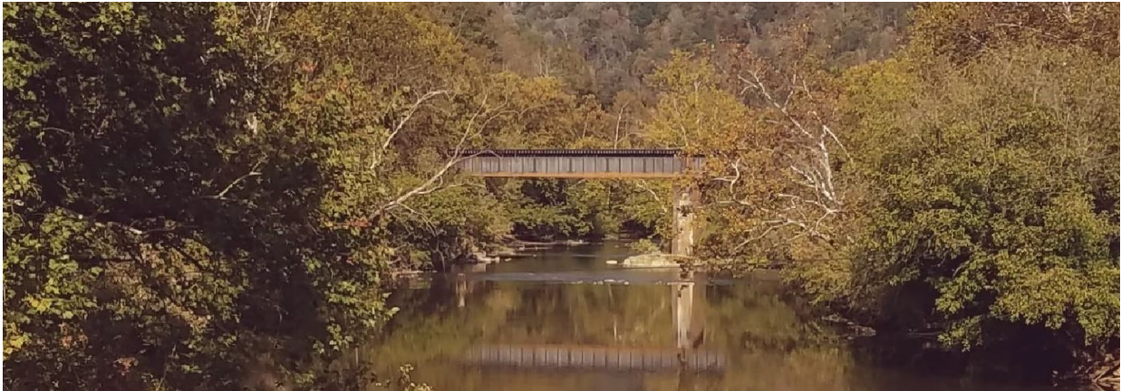
Figure 28: Photograph of Railroad Bridge over Clinch River near Artrip, Virginia
