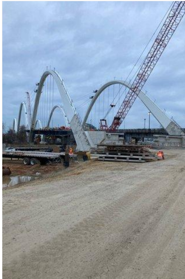
Frederick Douglass Memorial Bridge under construction.
