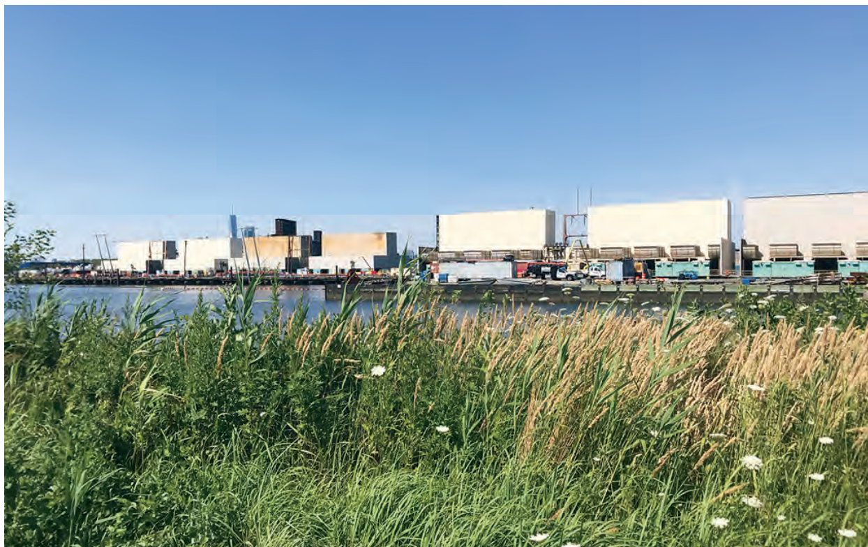
Gowanus gas turbine facility peaker in Brooklyn. PHOTO: NEW YORK LAWYERS FOR THE PUBLIC INTEREST
