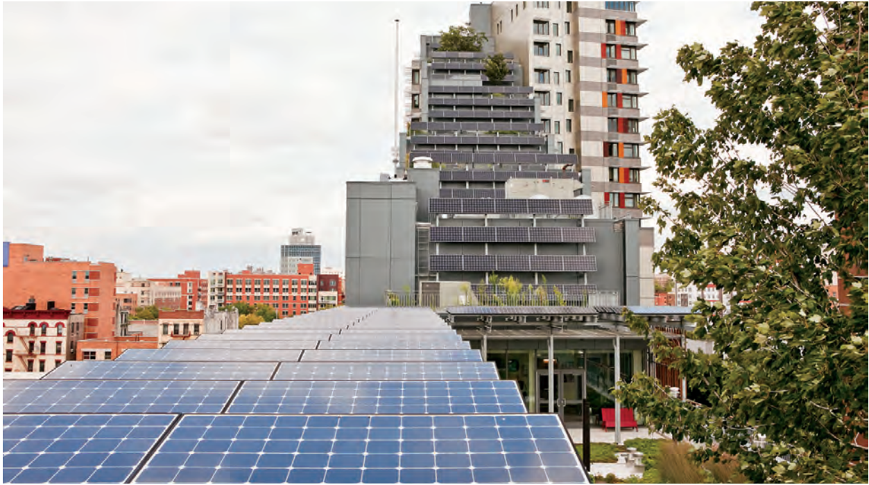
Via Verde housing development showcasing clean energy technologies in The Bronx. PHOTO: BRIGHT POWER
