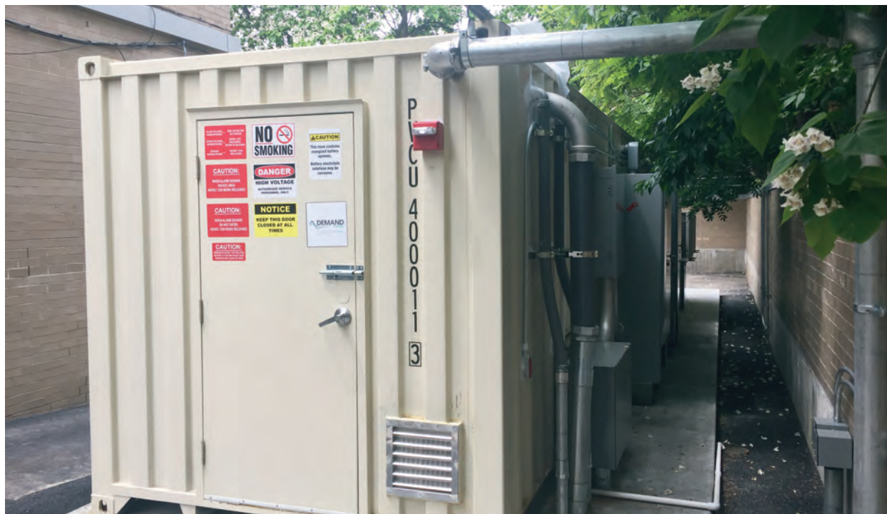
Battery storage installation that is paired with rooftop solar at Marcus Garvey Apartments affordable housing complex in Brooklyn. PHOTO: ENEL X
