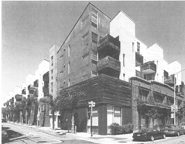
Construction of Folsom & Dore Apartments, which houses 130 low-income individuals, including those with a history of homelessness, benefited from reduced parking requirements.
