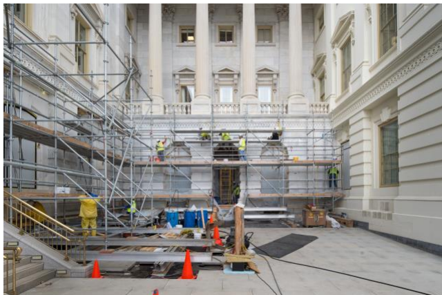
CAPITOL EXTERIOR STONE & METAL PRESERVATION PROJECT
