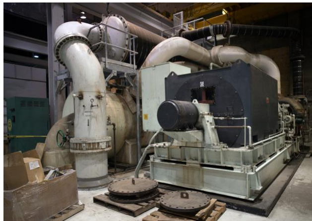
CAPITOL POWER PLANT REFRIGERATION PLANT REVITALIZATION PROJECT
