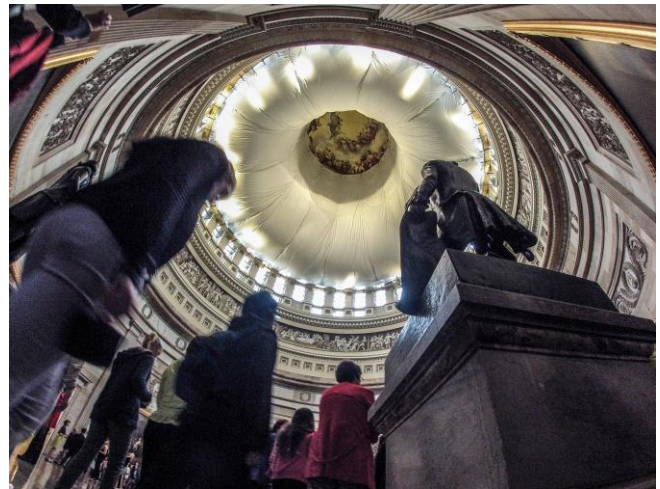
Safety canopy over the Rotunda in support of the Capitol Dome Restoration.
