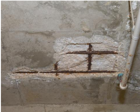
Deteriorated concrete slab in Rayburn Building Garage.
