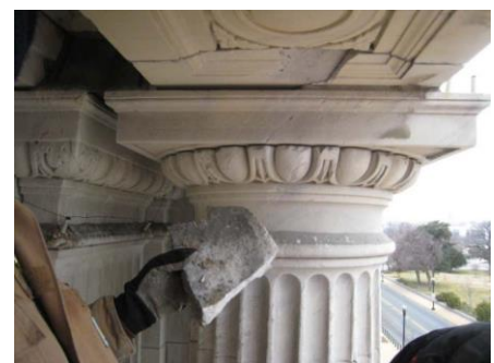
Deteriorating stone on the Cannon House Office Building exterior.
