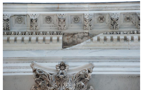
Spalling stone on the U.S. Capitol Building.
