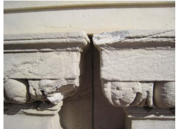
Spalling stone on the Cannon House Office Building.
