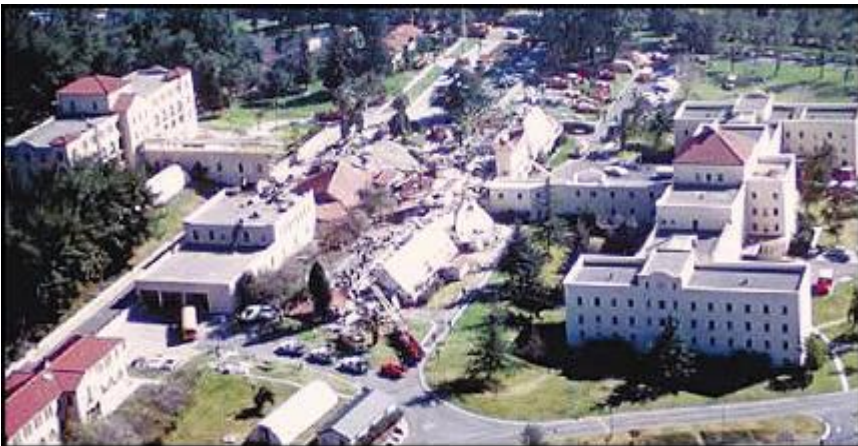
San Fernando Medical Center collapse, 1971
