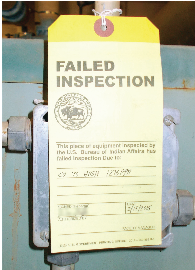
Figure 9: Failed Boiler Inspection Tag in a Bureau of Indian Education (BIE) School Classroom Building
