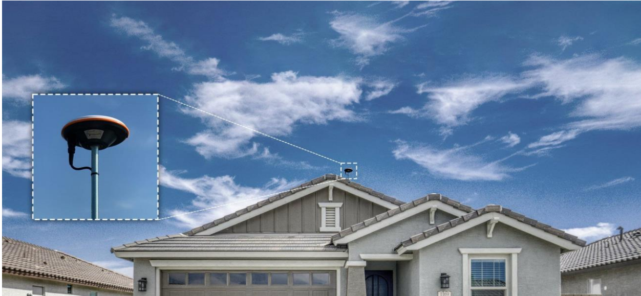
Image 2: Typical GEODNET Antennae Installation
