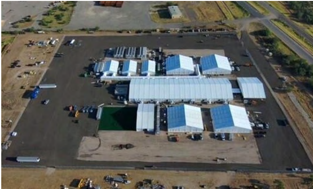
Figure 2. Soft-Sided Facility at Laredo, Texas
